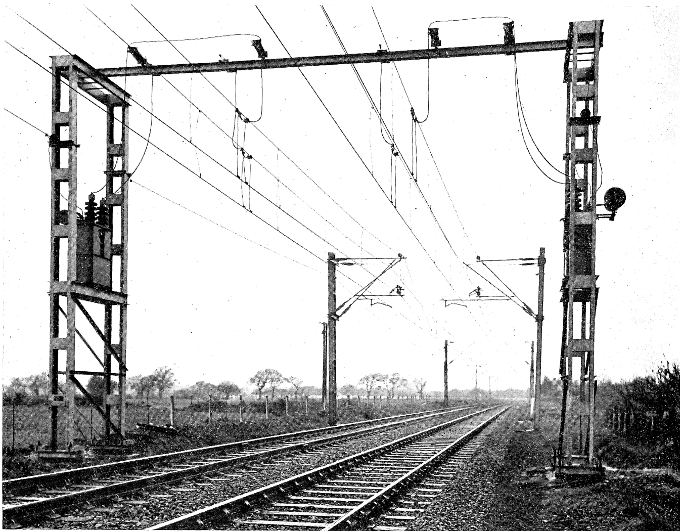
Fig.4 Booster Transformer mounted on structure
