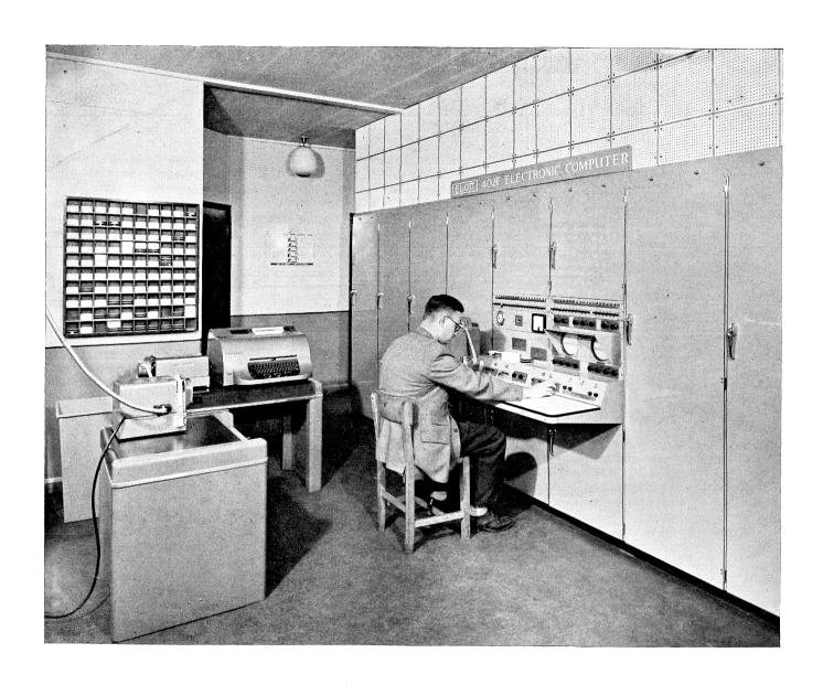
Fig.2 The British Railways research computer, with output printer
