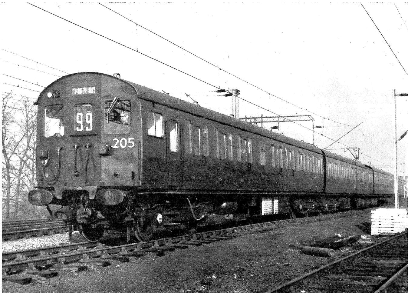
Fig.1 4-Car Unit, looking from B.D.T. end. London – Tilbury – Southend Line.
