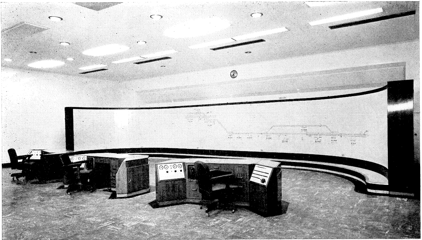
Fig.4 Crewe control room—Scenic diagram
