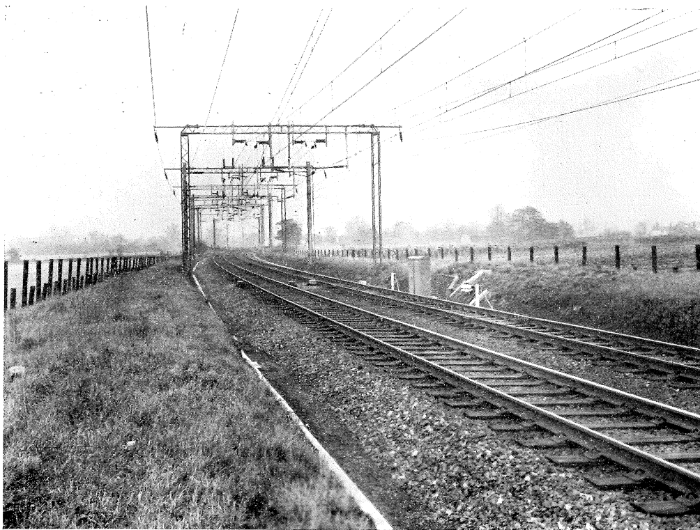
Fig.7 Carrier Wire Neutral Section
