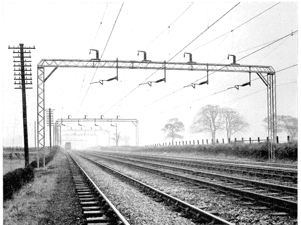
Fig.2 Catenary supporting insulators mounted above structure boom
