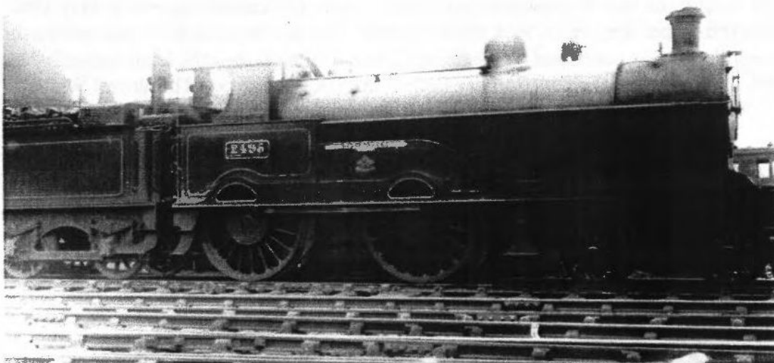
(DNR 721 - Large Boss Wheels on 'George the Fifth' No. 2495 BASSETHOUND : Mr C J B Cooke became Chief Mechanical Engineer in 1909 and soon revived Webb's concept of a large circular wheel-boss for his 'Georges'. Unlike Webb's completely symmetrical wheel, however, the 'George' version has a balance weight cast on the rim.)
