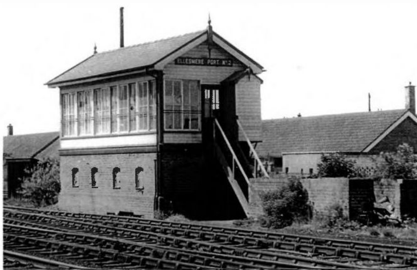
Ellesmere Port no.2 signal cabin. Opened about 1924 by the L.M.S.R./G.W.R. Joint Railway. It had an L.N.W.R. tappet frame of 45 levers. Closed by British Railways in November 1983. Photographed on 14 June 1975; (caption by John Dixon).
